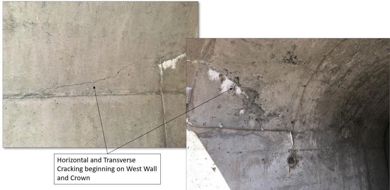
Photograph 6. Interior Cracking – West wall
