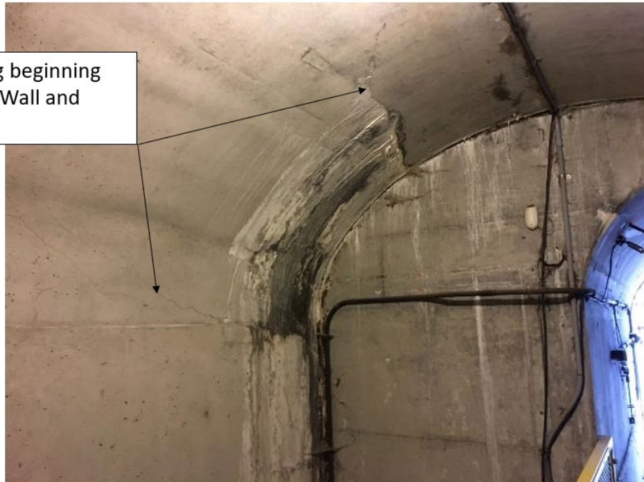
Photograph 8 – Cracking at Interior Chamber
